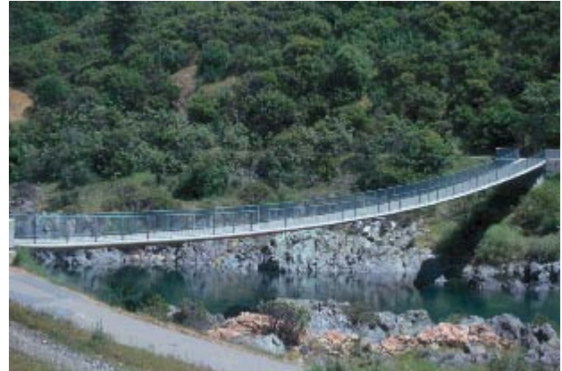
Stress Ribbon Bridge Across Sacramento River
