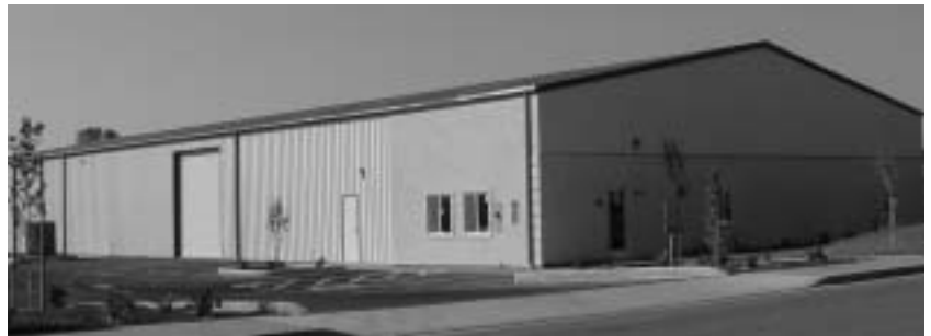
This photograph illustrates the lack of good street presentation given its unarticulated wall and roof forms and monotonous materials.
